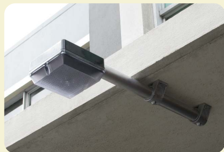
"Exterior light" sensor is used where there is no eave or overhang on which to mount a sensor.
